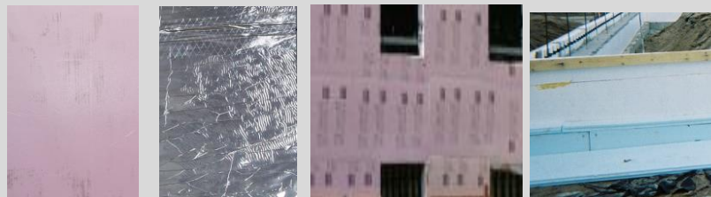
CI insulation (from left to right): XPS sheet, Polyisocyanurate sheet with foil facing, XPS over steel framed walls, EPS over concrete wall and foundation.
